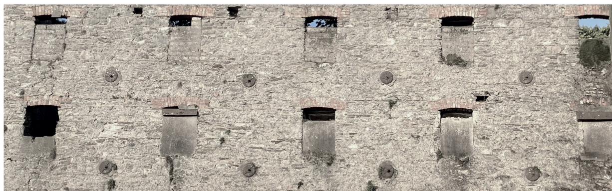
East wall, evidence of lime render on stone work details.
