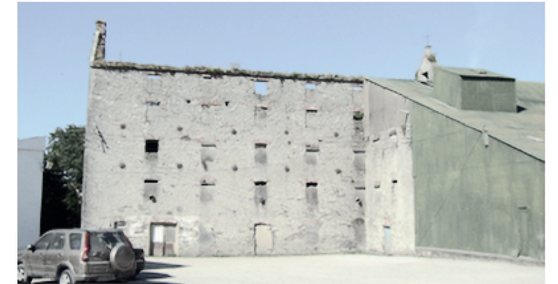
Figure 15: East elevation of the main structure.
