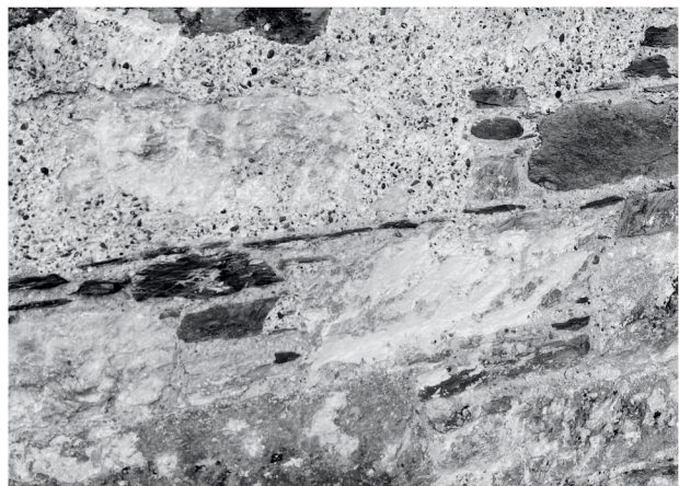
Figure 16: View of cobbled stone wall on the exterior.
