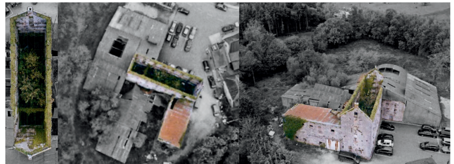
Drone aerial view footage of the mill structure within the Glenbower woodland:
