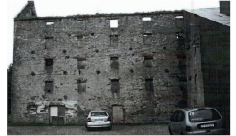
Figure 10: East elevation of the main structure.
