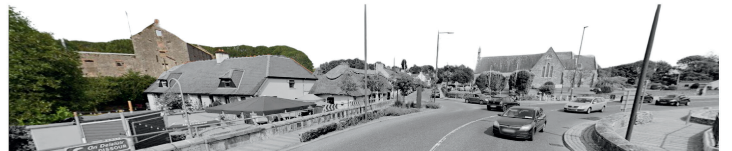
The mill structure is highlighted in the above image travelling east on the N25 Youghal road:
