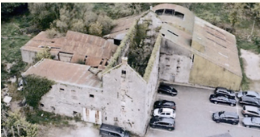
Figure 6 site context view from south gable.
