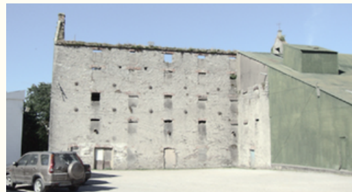
East elevation of the building.
